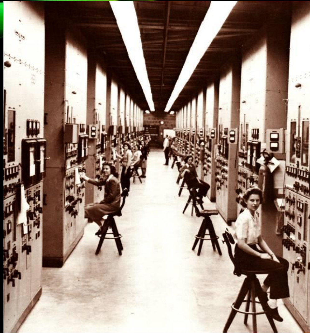
Control panels and operators for calutrons at Oak Ridge. The operators, mostly women, worked in shifts covering 24 hours a day.
