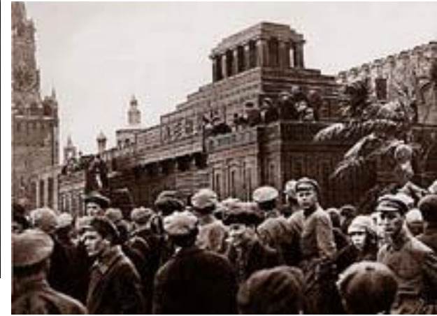
Temporary Mausoleum, Red Square, Moscow, 1924
